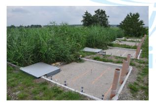
Figure 4: A media-based constructed wetland showing planted and unplanted treatment cells. (http://www.cenews.com/magazine-article----designing treatment wetlands for the 21st century-8517.html)
