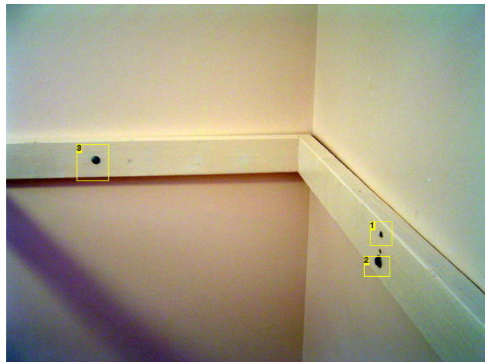
Image Notes 1. I used a deck screw to pin the frame in place temporarily... 2. ...before adding the lag screw. 3. These MUST go into studs
