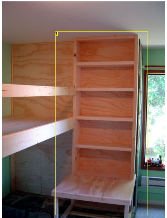
Image Notes 1. Bookcase, six shelves. The second one down was placed to line up with the top of the rail - the rest are spaced with gaps that I thought looked about right
