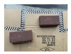
3) Apply primer to bricks with painter brush (**WARNING**: If step is skipped, will result in paint not sticking to brick and sinking into brick)
