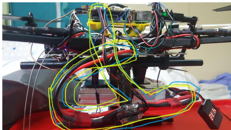
The power from battery splits through the power module to the power distribution board and Navio2
