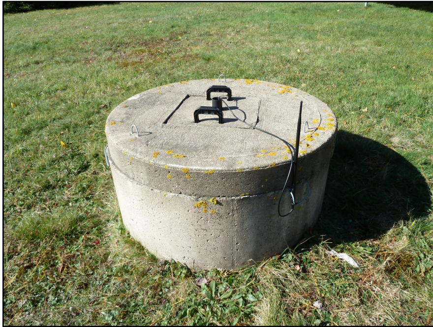
Figure 11: External antenna on side of well with cable leading to meter inside well.
