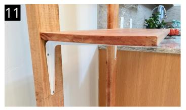
Place the desk back onto the shelf brackets and use screws to fasten.
