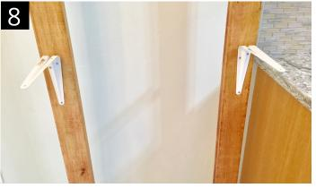
Mark a spot 100cm (40") from the floor. Fasten the 7" x 9" shelf brackets to the post.
